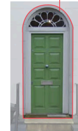
Beaded panel door with rectangular fanlight and gabled hood
