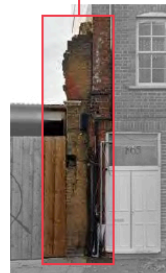
Retained portion of arched entrance to neighbouring plot
