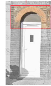
Original brick arch over front door
