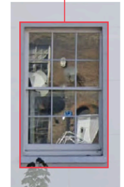
Recessed sash windows
